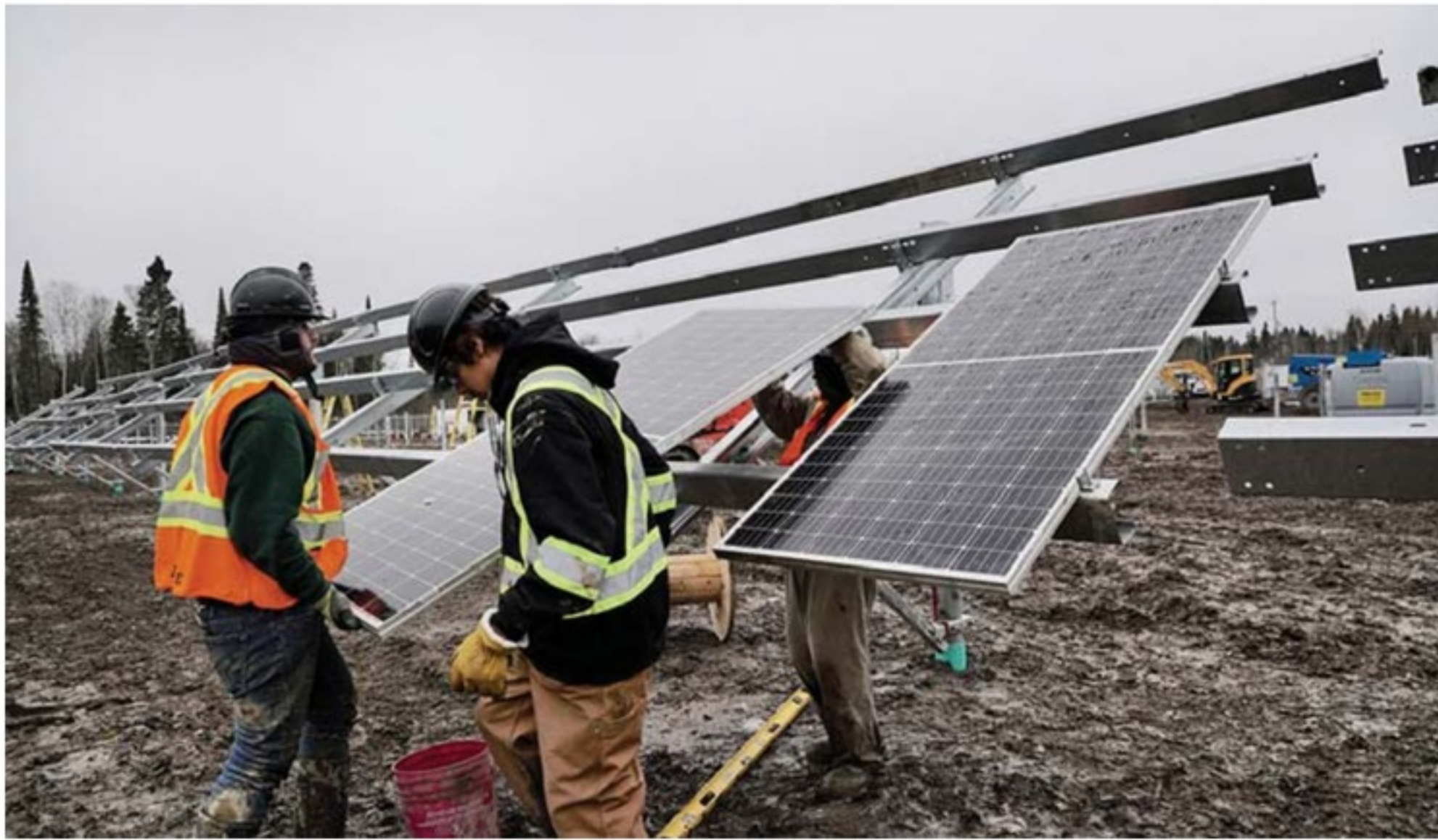
Assembling photovoltaic solar panels.
